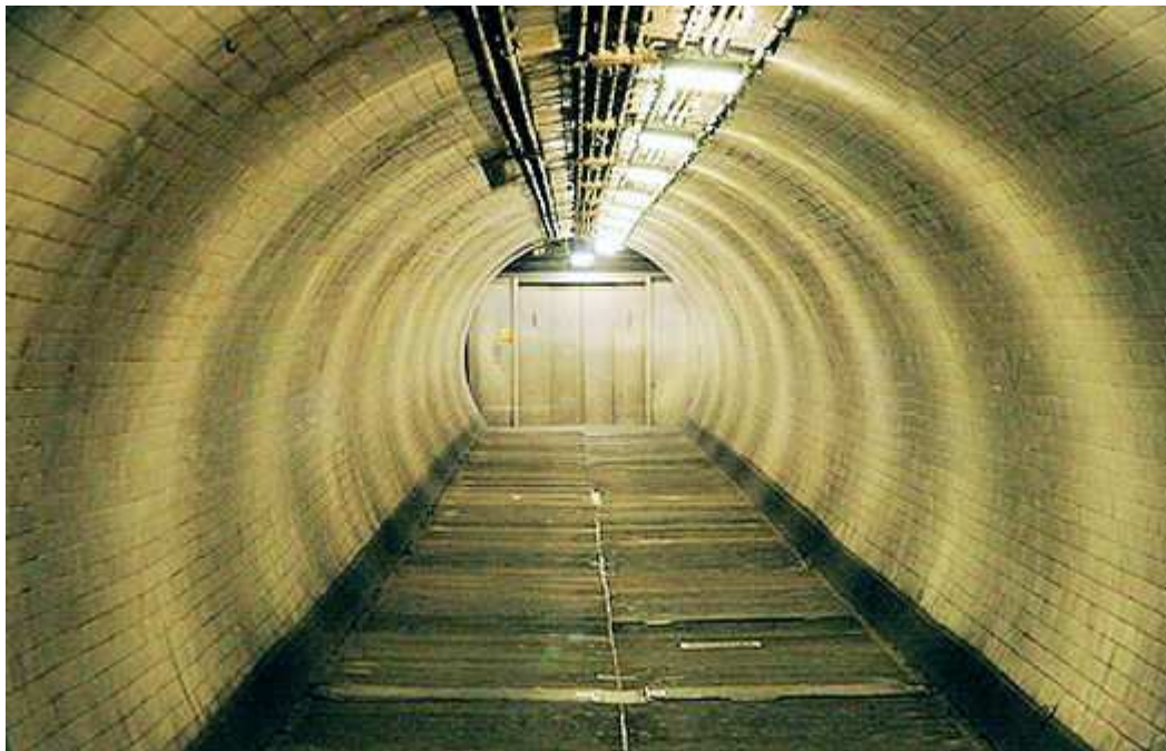
Inside the Foot Tunnel
